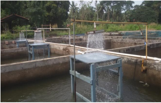
Wooden perforated sheet aerator
