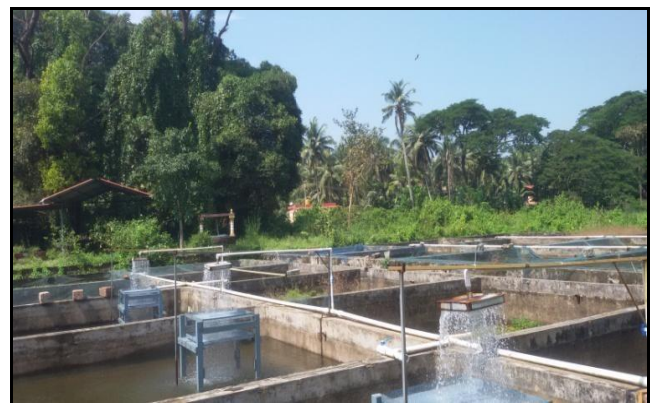
Two Tier Perforated Sheets Aerator
