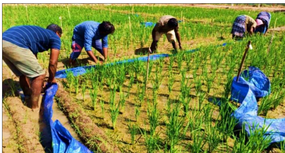
Fig 1: Inserting polythene sheets on all four sides of the plots to prevent water seepage
