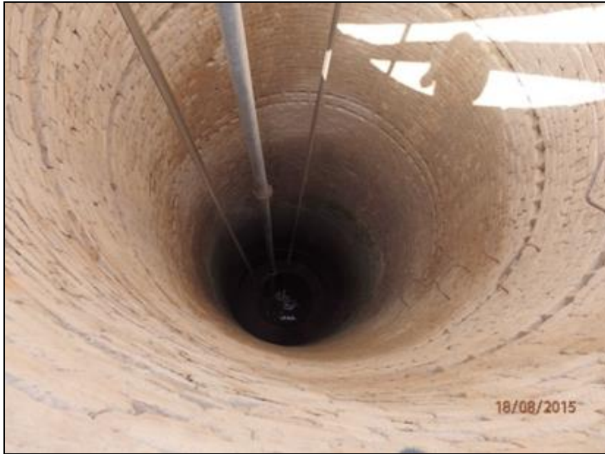
Fig 7: Over-depleted well with high pumping cost in District Vehari, Punjab, Pakistan
