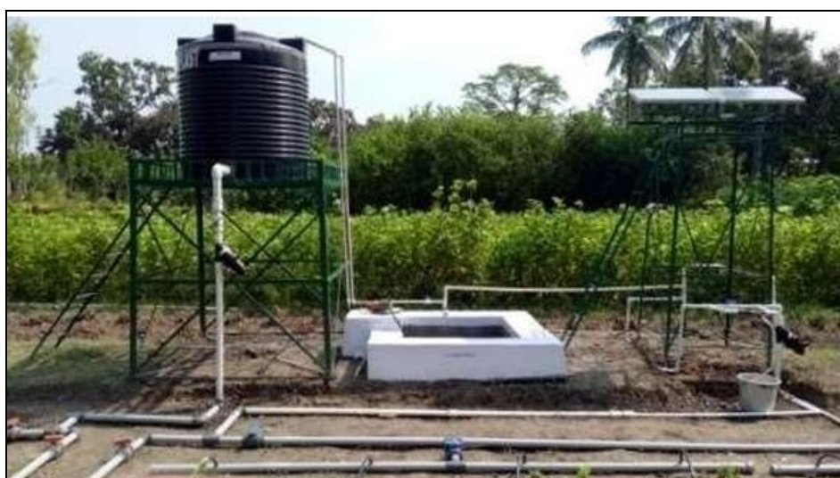
Fig 1 (a): Solar drip irrigation kit with two solar photovoltaic panels (80 Wp)
